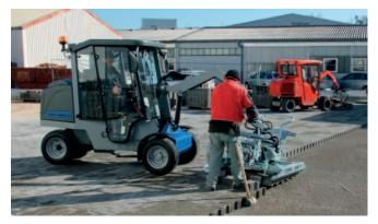
Six hours of paver installation – smooth running, low noise and no exhaust fumes. The world's first fully electric laying machine is designed for endurance. It is also of particular advantage when used in areas with stricter limits for exhaust and noise emissions, e.g. in underground car parks or near hospitals and schools.
