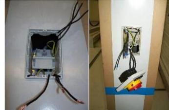
9. Insert the mounting frame into the crane column and guide the cables out before the frame is permanently fastened. Screw the mounting frame to the column using the clips that are provided and then install the sealing. Connect the main switch Set the motor protection switch to the rated value of the motor
