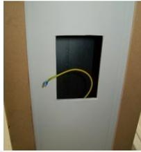
1. Attach the ground cable to the inner side of the crane column using nuts and the washers that are included with the crane column.
