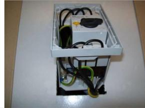
7. Push the cables back through into the column and place the mounting frame into the crane column. Then screw the mounting frame to the column using the clips that are provided.
