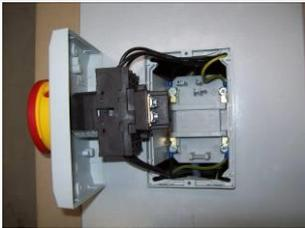
10. Then place the cover onto the mounting frame and screw it on.
