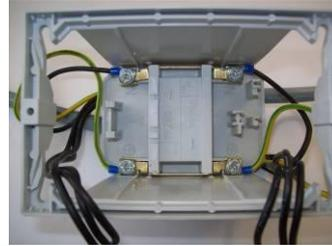
7. Connect the neutral and ground cables to the mounting frame
