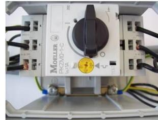
3. Connect the neutral and ground cables to the mounting frame and press the motor protection switch into the mounting frame and connect it.
