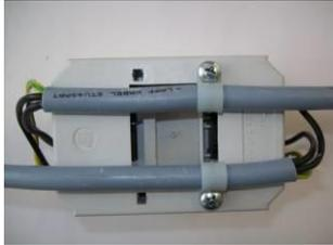
8. Lay the cables back around the mounting frame and secure them using the cable clamps.
