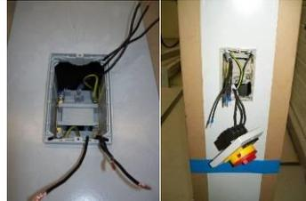
9. Insert the mounting frame into the crane column and guide the cables out before the frame is permanently fastened. Screw the mounting frame to the column using the clips that are provided and then install the sealing. Connect the main switch Set the motor protection switch to the rated value of the motor
