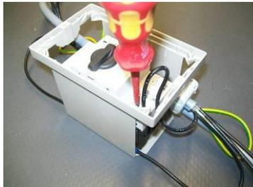
4. The motor protection switch has spring terminals. Use a small screwdriver for these, as shown in the illustration. The terminal opens when pressed down, and the cable can be inserted into this opening.
