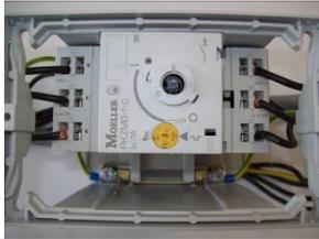
6. Remove the black rotary knob from the motor protection switch. To do this, carefully place a small screwdriver under the knob and lift it off.
