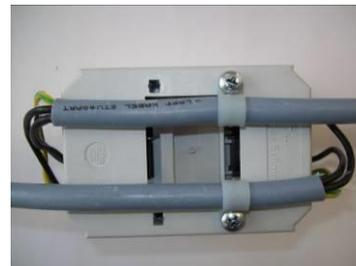
5. Lay the cables back around the mounting frame and secure them using the cable clamps.
