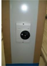
9. Place the cover onto the mounting frame and screw it on.
