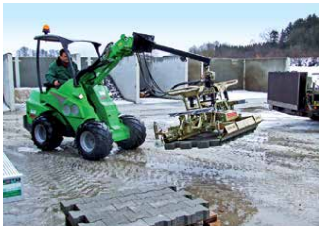
Installation clamp in combination with Mini-excavator
